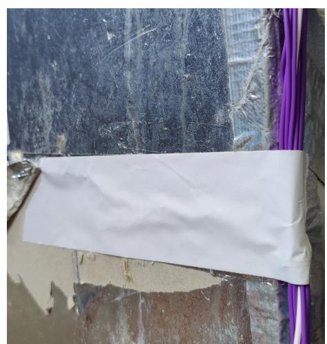
**Step 3:** Secure the loom at the rear of the fridge at both the bottom and top using foil tape, ensuring the loom does not protrude past the sides of the fridge and remains on the rear surface.
