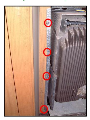
The units are usually held in by up to 4 screws on each side. Remove the screws and retain for refitting
