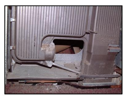
Remove the pipe clip and gently pull the pipe back through the hole shown above
