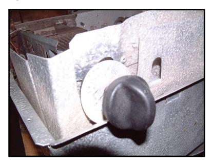
Fold back the half round metal tab so that you can release the gas control shaft and knob. Also unplug the electrical connector (with green and white wires) from the gas control unit.
