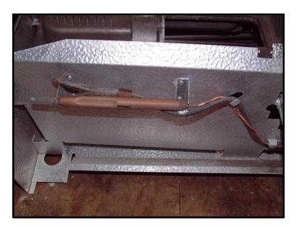
Release the two clips holding the thermostat bulb. Bend the cable retaining clips out so you can remove the thermostats/bulb with the heat exchanger. Bend them as little as necessary to avoid breaking them off.
